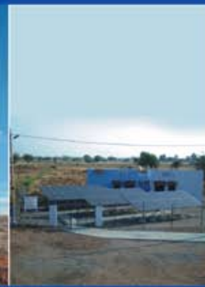
Off Grid System
